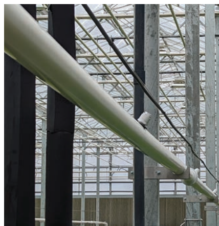
Co2 is safely distributed through nozzles.
