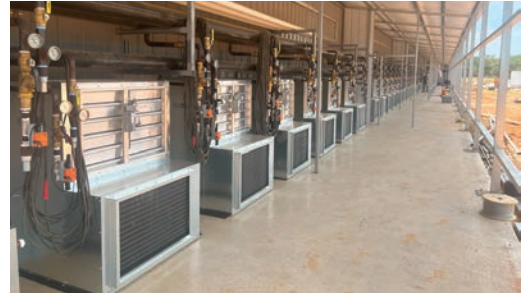
Air handling units with a bypass at Compassionate Cultivation, a medicinal cannabis facility in Bastrop, TX.
